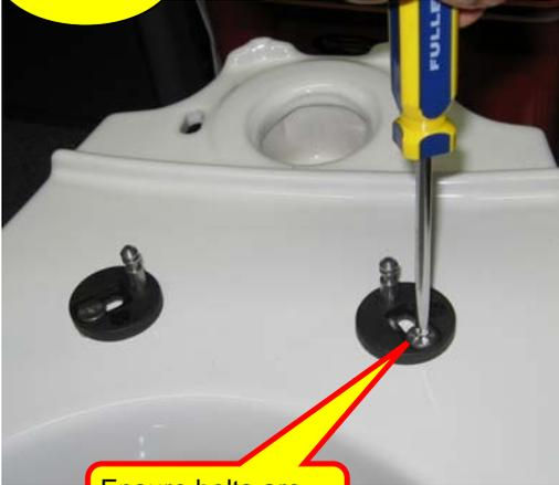
Ensure bolts are fully tightened
