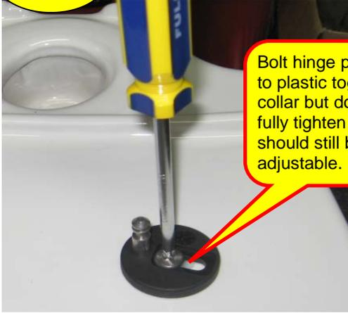
Bolt hinge plate to plastic toggle collar but do not fully tighten - it should still be adjustable.
