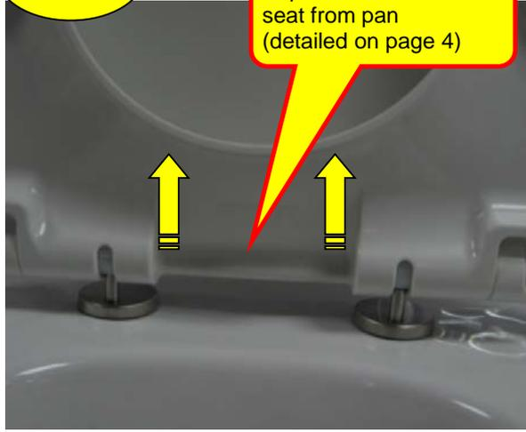
Separate and remove seat from pan (detailed on page 4)
